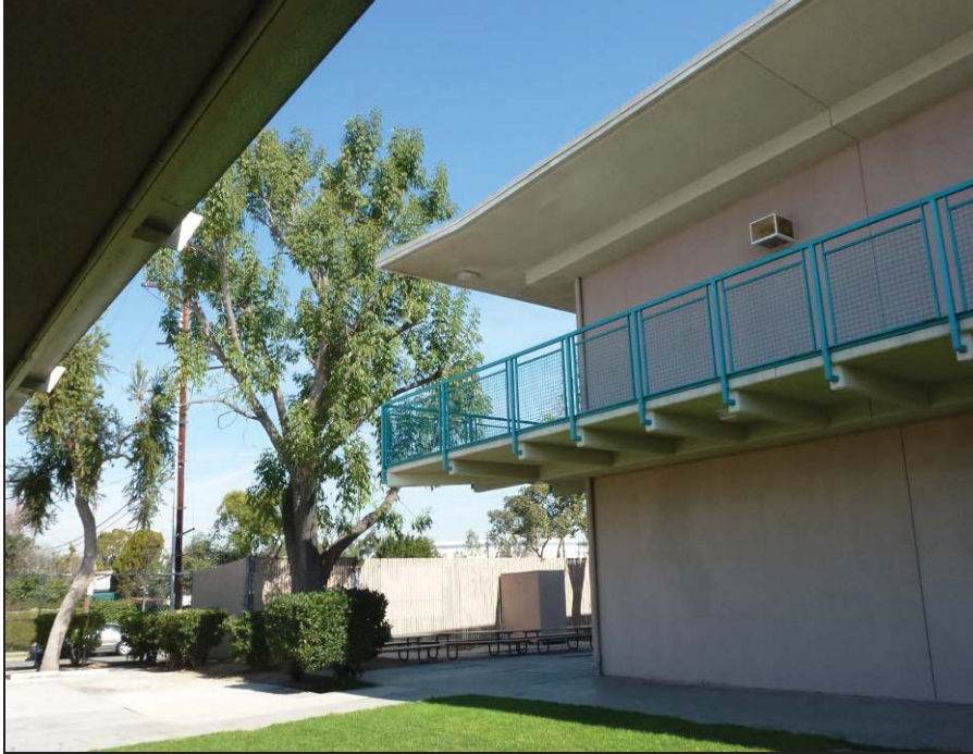
Leapwood Avenue Elementary School, Classroom building showing wide overhang with folded plate. Source: Sapphos Environmental, Inc., 12 February 2014.
